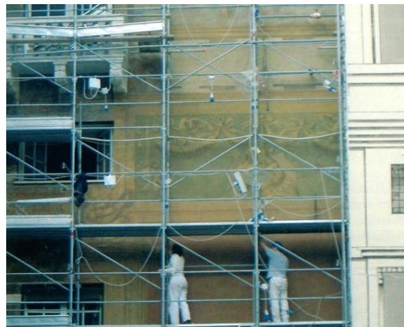
Façade restorations to Palazzo Doria Spinola (source: ARKOS Speciale G8, 2001).
